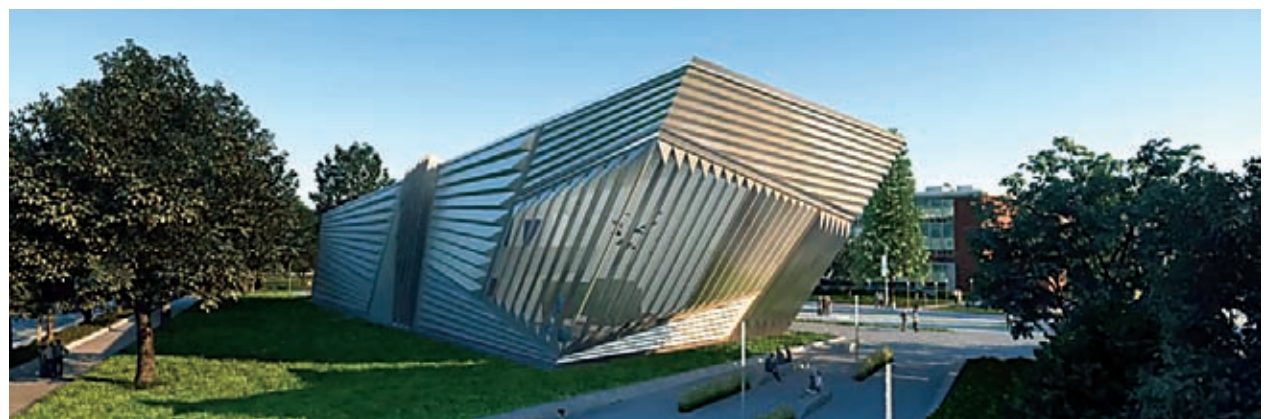
A view of the planned Eli and Edythe Broad Art Museum from the northwest. Courtesy of Zaha Hadid Architects.
